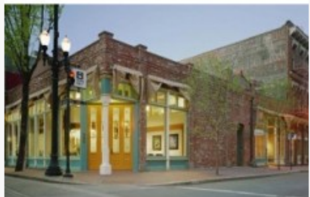
HISTORIC RECONSTRUCTION IS GOOD: A recent renovation of the 1885 Freimann Building in the Skidmore Historic District of Portland, OR, involved removal of its 1960s remodeled front (top image) and total re-creation of the original façade's contours and details. Some preservation purists would call this "false history." But the new HPLO report shows that – more importantly – the historic reconstruction helps re-establish the overall special character of the district. Photos: Architectural Heritage Center, Portland, OR
