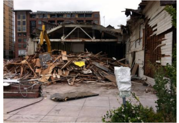
Demolition of a contributing building, 2011
