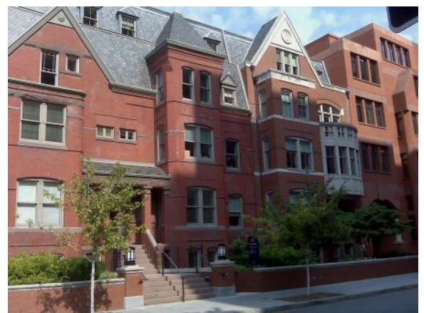
Two distinct approaches to infill over time. The original historic building is on the left.
